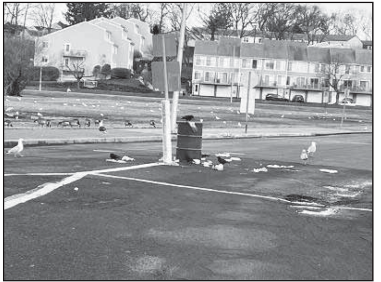
Potholes are a problem all over the city at this time of year, and many complaints have been received concerning overflowed trashbins at the bike/walk path. Here are two examples.
