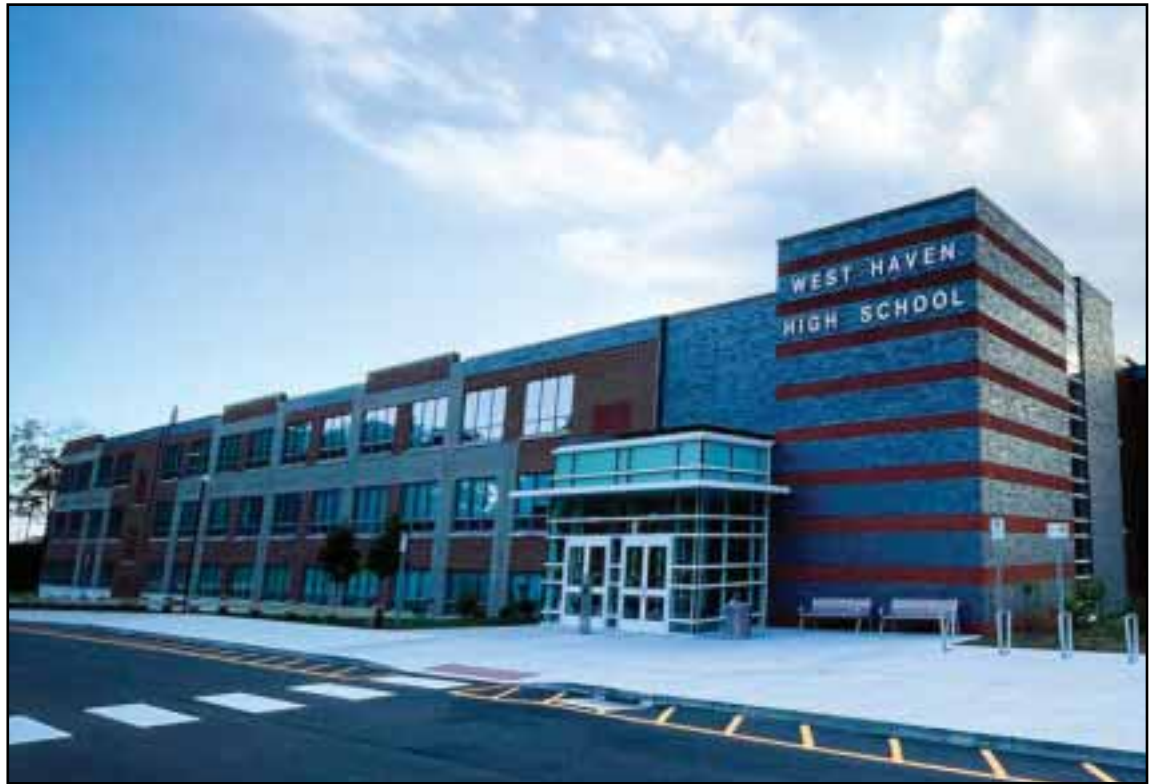
The two-year-old West Haven High School was awarded by the Connecticut Building Congress for its "team effort" in rebuilding the 1963 structure. The $130 million project came $2 million under budget, with several unplanned additions during construction.
