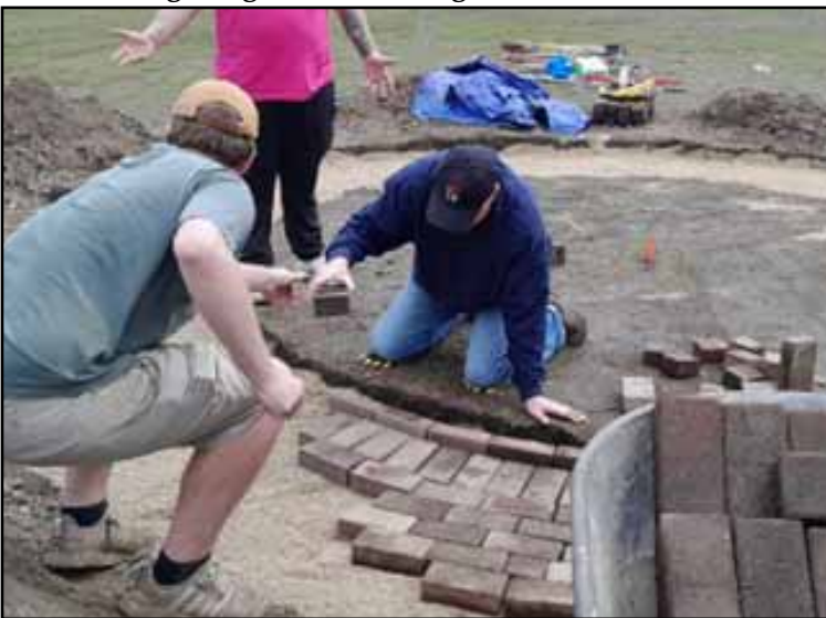
Scouts and other volunteers lay the bricks that make up the outer ring of the garden.
